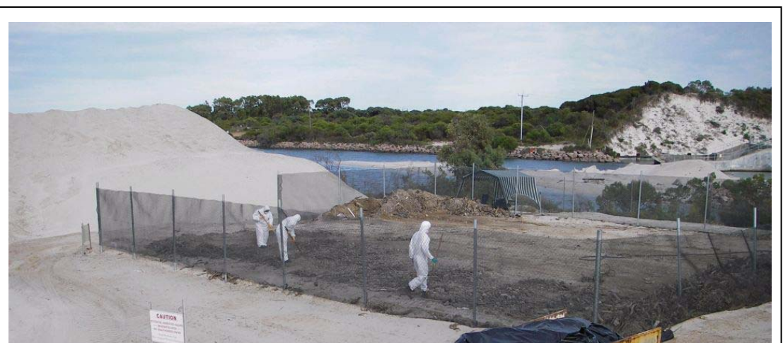
Raking of surface soils to remove ACM fragments
